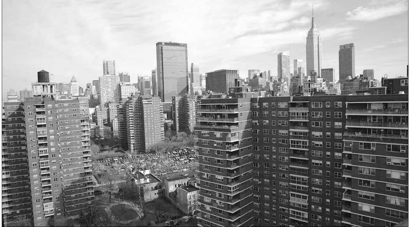
Penn South is 10 buildings with 2,810 apartments in the heart of Chelsea.
